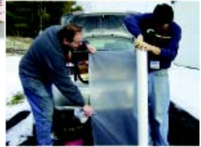
RIGHT: Volunteers cut plastic sheeting to be placed around the base of a mobile home. The plastic prevents drafts from entering the base of the home.
